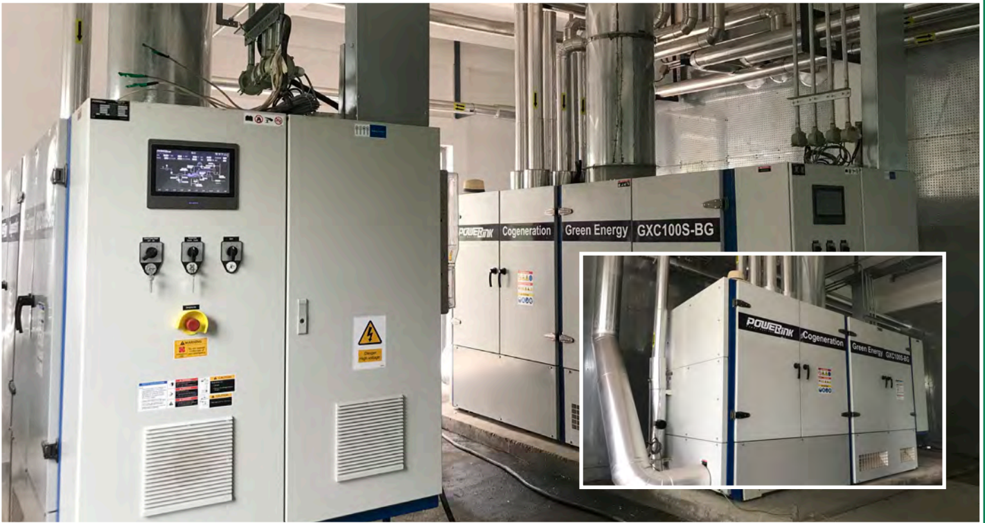
Agriculture Biogas Cogeneration Application 100KW
